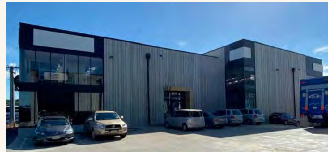
NEW ZEALAND WAREHOUSE
