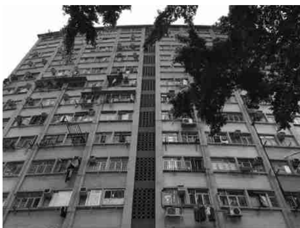
Exterior of the subject building – On Ning Building
