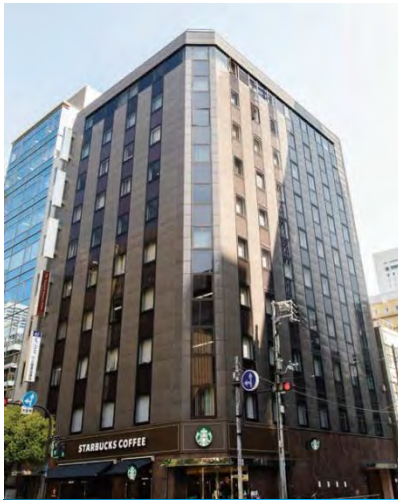
Yotsubashi East Building
