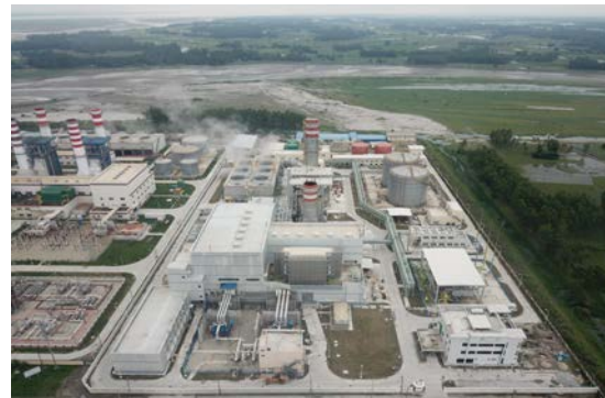
The Sirajganj Unit 4 combined cycle gas turbine power plant in Bangladesh commenced commercial operations in 2019
