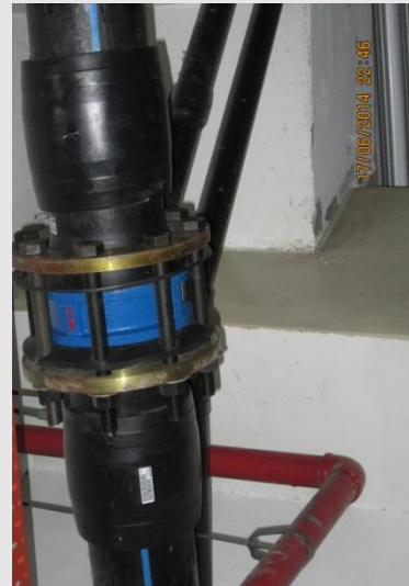
New Flood Mitigation Pump
