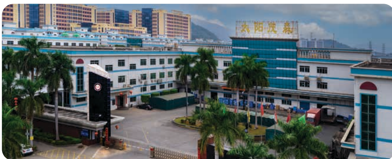
▲ Sun Mansfield Plant
