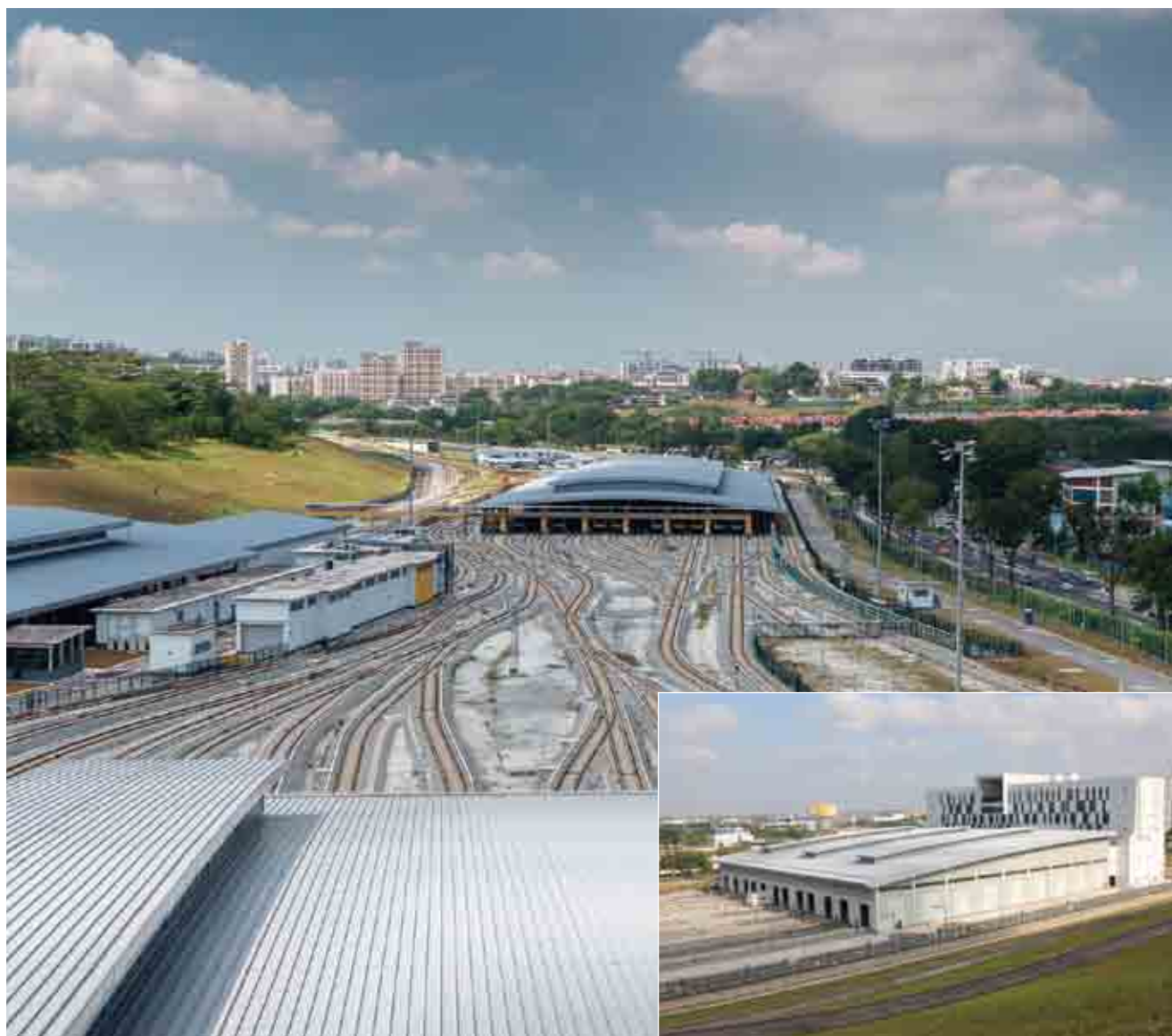
Civil Engineering Jalan Gali Batu Depot Project
