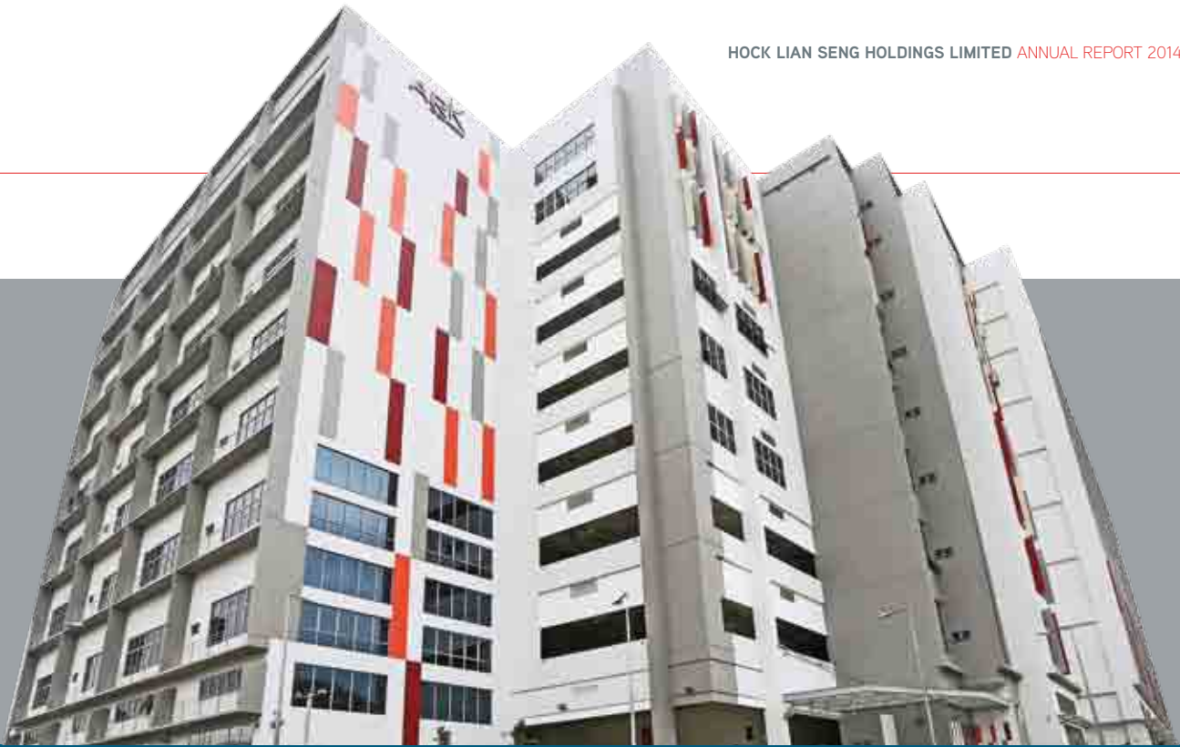
ARK@GAMBAS COMPLETED IN 2014
