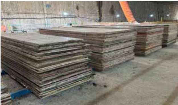
Plywood is recycled for formwork.
