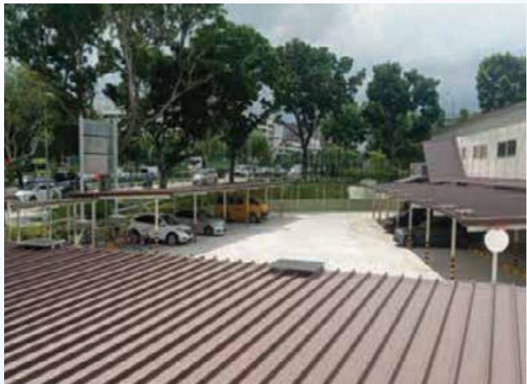
Site office solar Energy light
