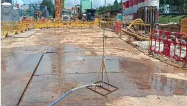
Portable water sprinklers are used for dust control.
