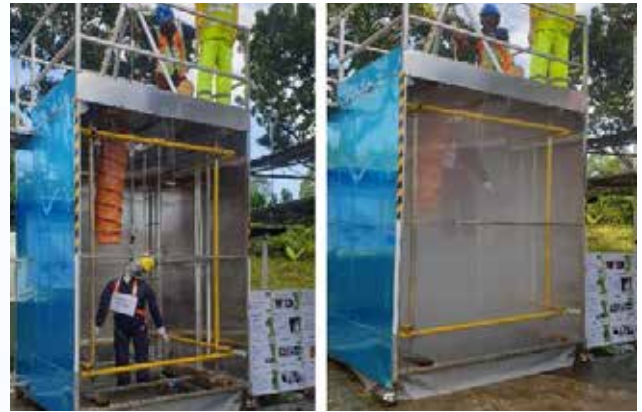
Training on entry into and rescue from confined space.
