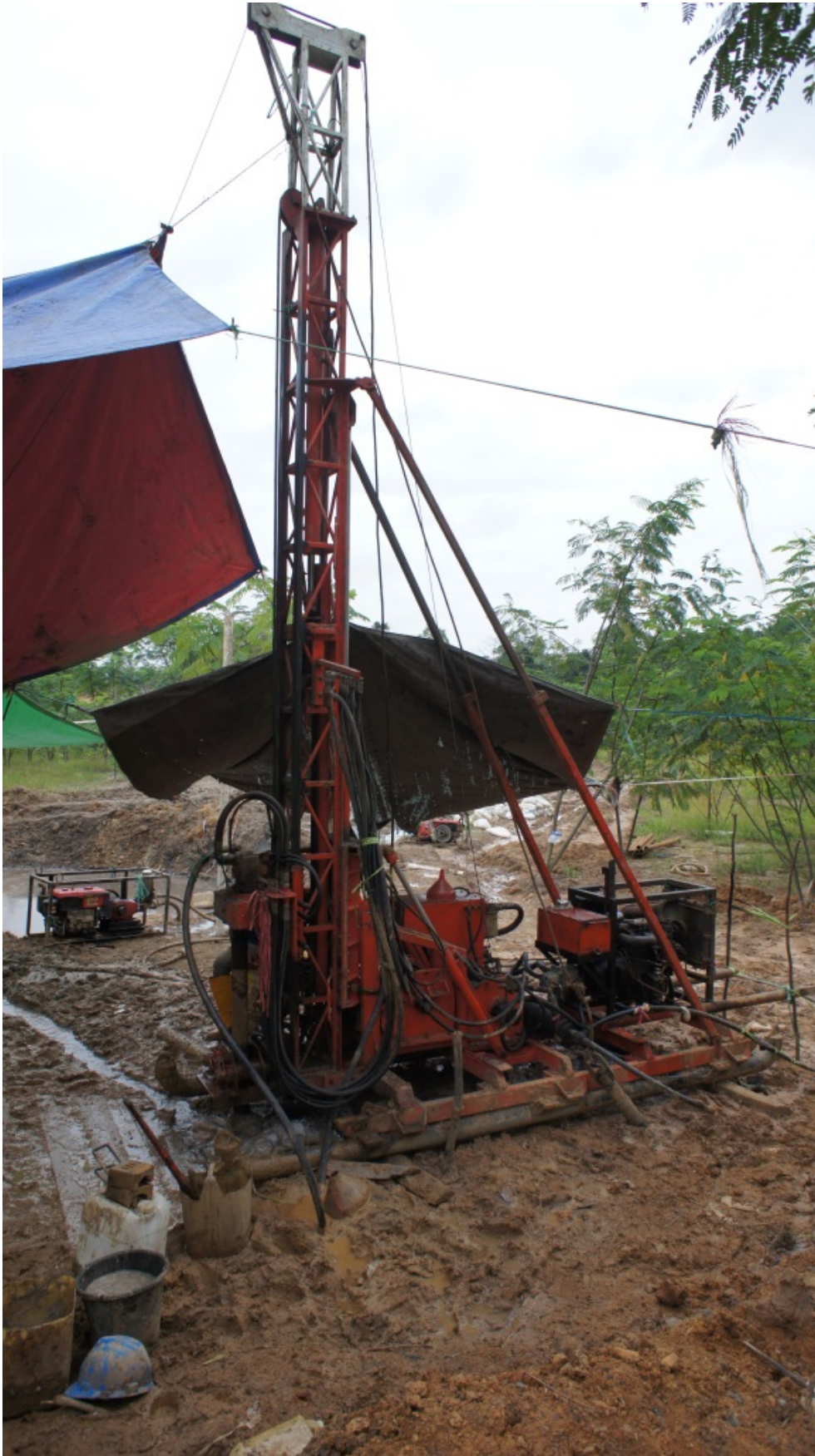
Figure 4.1 – Drilling Rig at RK
