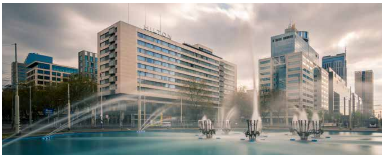
Hilton Rotterdam Hotel, Rotterdam, the Netherlands
