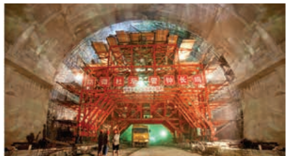
One of the largest cross-section cuts in Asia – underground construction of Chongqing Rail Transit Line 6 - Jin Shan Si Station (two-layer train station with 307 m 2 section excavation area)
