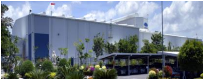
Metal coating & painting facility, Map Ta Phut
