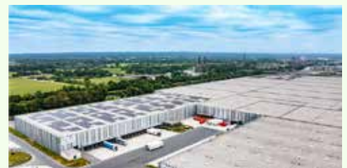
Goodman's largest solar installation globally Marl, Germany
