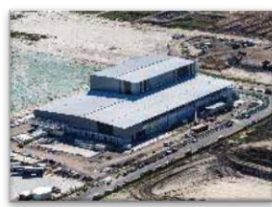
Corner Heron Drive and Curlew Street, Port of Brisbane
