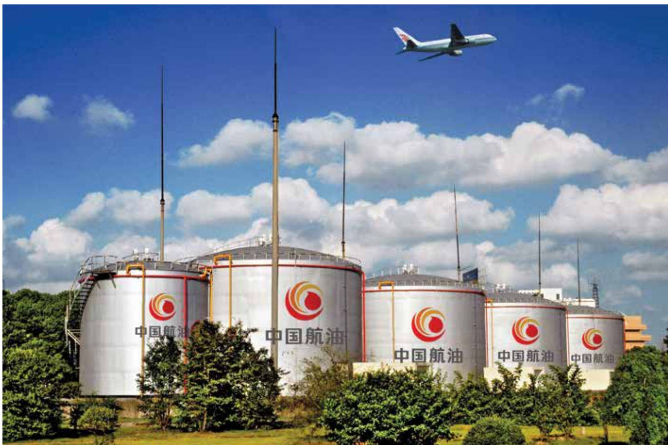
CNAF storage tanks in the PRC CNAF在中国的储罐
