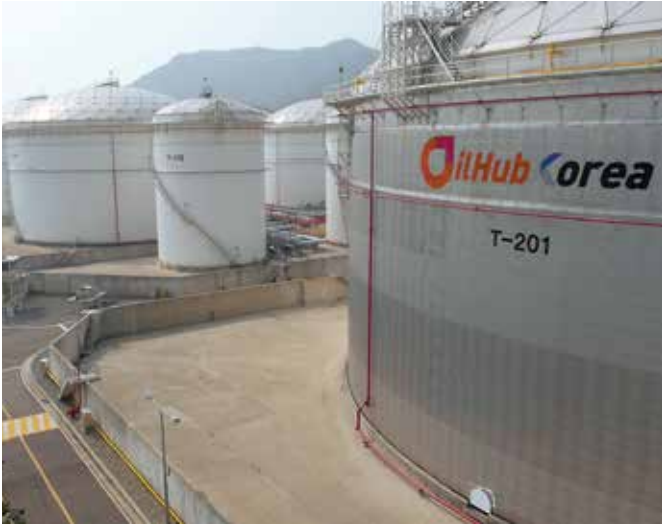
OKYC storage facilities OKYC的储罐设施
