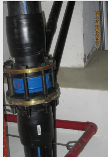
New Flood Mitigation Pump
