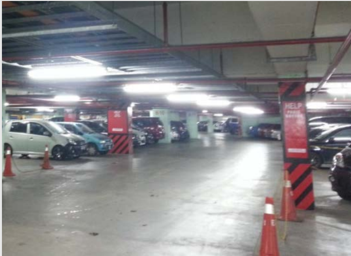
New T5 Lighting at Basement Car Park
