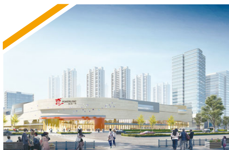
ZHUHAI GAOXIN POWERLONG PLAZA
