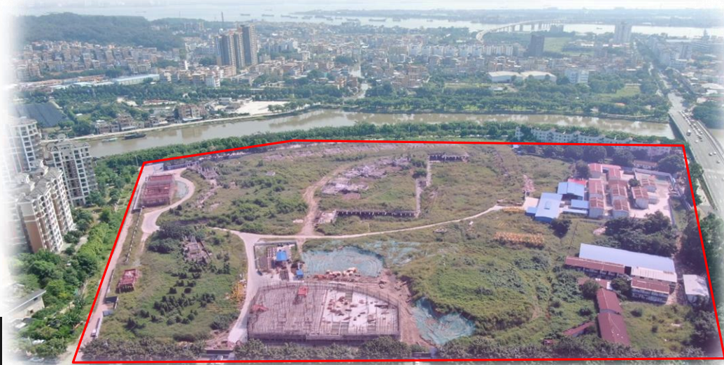
Phase 3 of Le Papillon project in Panyu, Guangzhou
