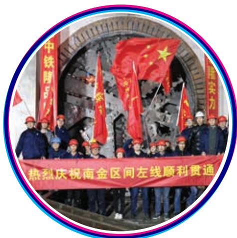
Ningbo Metro Line 4 – Successful tunnelling
