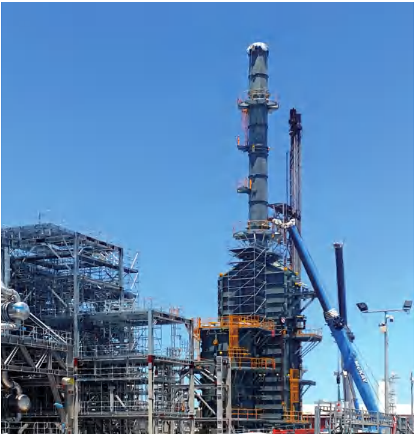
Direct-fired process heater system at O&G refinery, Australia
