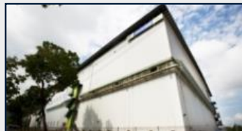
2 ALOG Cold Centre 2 Fishery Port Road
