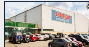
19 217 – 225 Boundary Road, Laverton North
