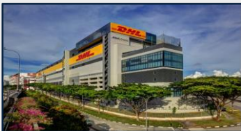
10 DHL Supply Chain ARC 1 Greenwich Drive
