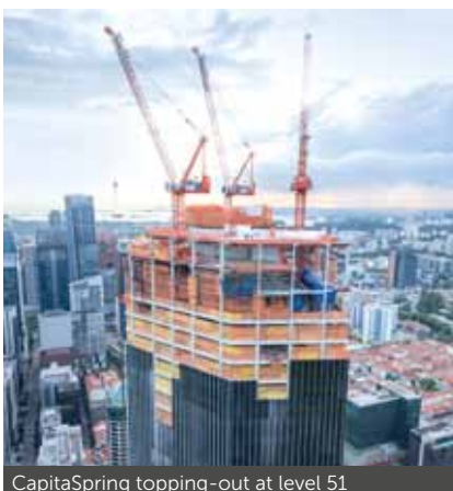
CapitaSpring topping-out at level 51
