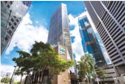
4 Six Battery Road
