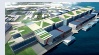
Datapark+ Scalable and efficient modular data centre park
