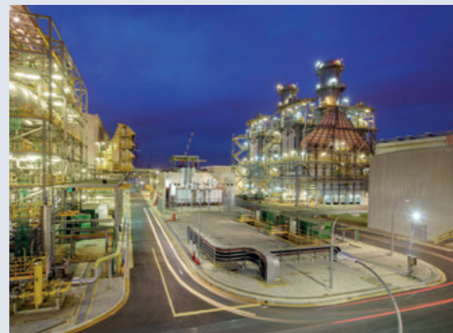
Keppel is a strong operator with a track record for engineering, developing and operating specialised assets, including Keppel Merlimau Cogen, a 1,300 MW Combined Cycle Gas Turbine power plant in Singapore.
