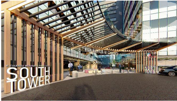
New and extended canopy and passenger drop-off area 1
