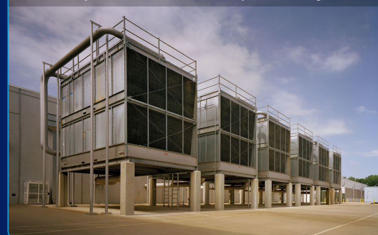
Concurrently Maintainable Chillers, Pumps and Cooling Towers
