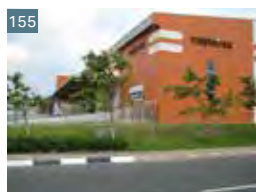
155 Mapletree Logistics Centre
