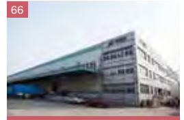
66 Mapletree Northwest Logistics Park (Phase 2)
