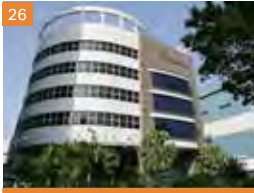
26 3 Changi South Lane
