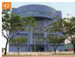
42 73 Tuas South Avenue 1
