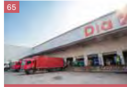
65 Mapletree Northwest Logistics Park (Phase 1)
