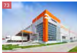
73 Mapletree Tianjin Wuqing Logistics Park
