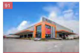
91 Mapletree Changsha Airport Logistics Park
