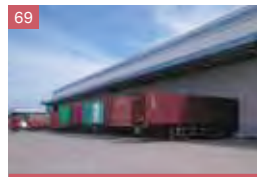
69 Mapletree Yangshan Bonded Logistics Warehouses
