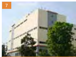
6 Changi South Lane
