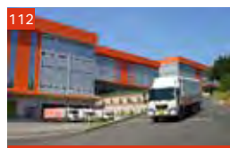
112 Mapletree Logistics Centre – Iljuk
