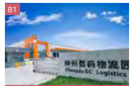
81 Chengdu DC Logistics Park
