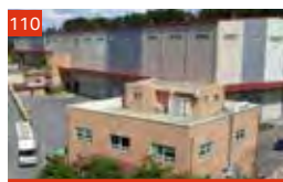
110 Mapletree Logistics Centre – Yeosu
