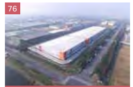
76 Mapletree Hangzhou Logistics Park
