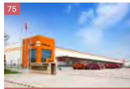
75 Mapletree Nantong Chongchuan Logistics Park
