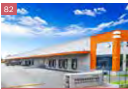
82 Mapletree Shenyang Logistics Park
