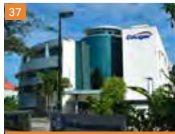
37 30 Boon Lay Way
