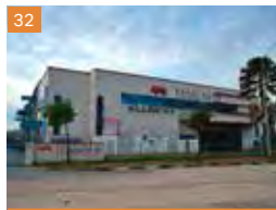
32 30 Tuas South Avenue 8
