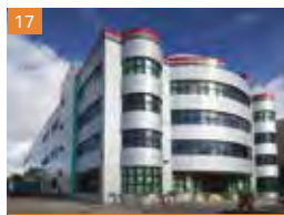
39 Changi South Avenue 2
