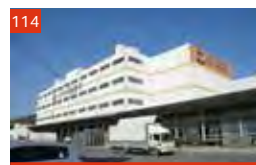
114 Mapletree Logistics Centre – Anseong Cold
