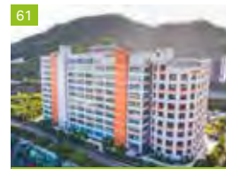
Mapletree Logistics Hub Tsing Yi
