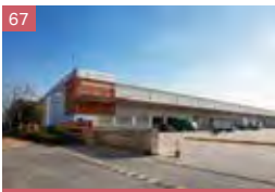
67 Mapletree (Wuxi) Logistics Park
