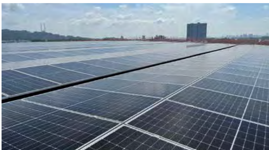
Solar panel installation at Mapletree Logistics Hub, Toh Guan, Singapore
