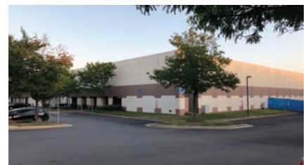
65 45901-45845 Nokes Boulevard, Northern Virginia, Virginia
