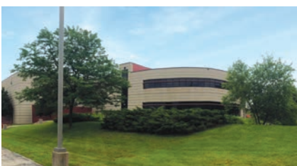
72 N15W24250 Riverwood Drive, Pewaukee, Wisconsin
