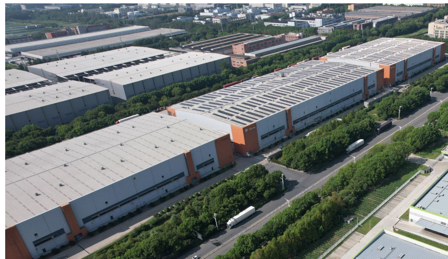
Rooftop solar installation at Mapletree Hangzhou Logistics Park.
