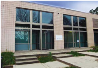
29. 1400 Cross Beam Drive, Charlotte
