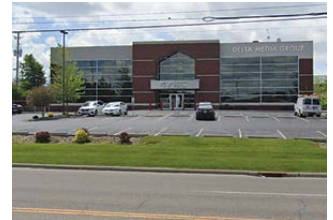
32. 4726 Hills and Dales Road NW, Canton
