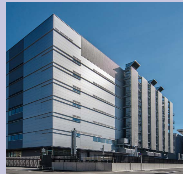
Osaka Data Centre ranked A under the CASBEE New Construction certification in July 2025
