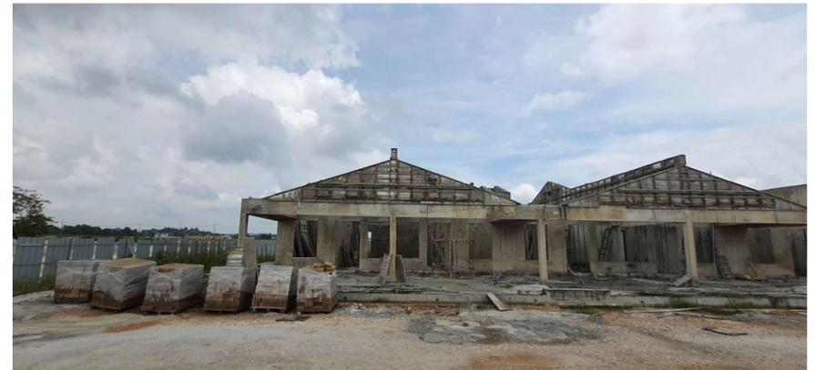
*Block 3A/B: Gable wall formwork installation in progress*
