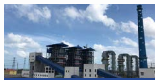
SHANTOU PROJECT (Phase 1)
