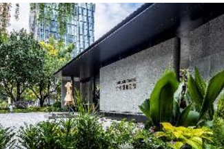
Yanlord International Apartments, Tower A, Nanjing 仁恒国际公寓, A栋, 南京
