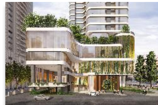
Yanlord Century Mansion, Shenzhen 仁恒世纪大厦, 深圳
