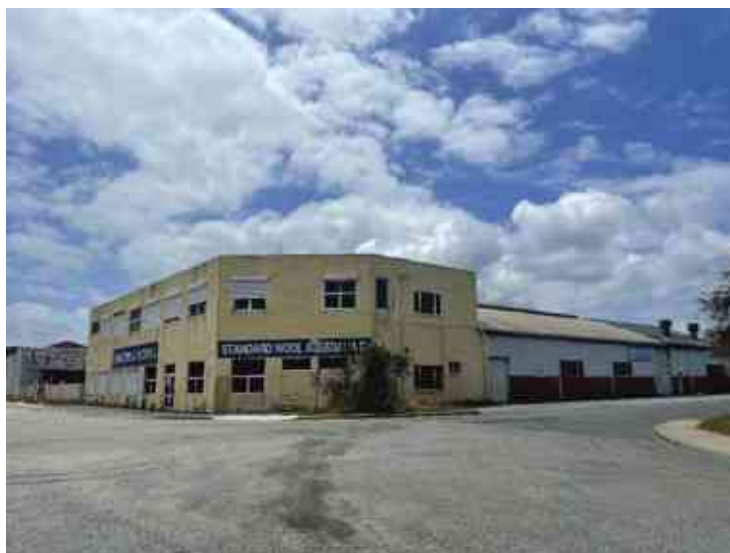
Former SWA site
