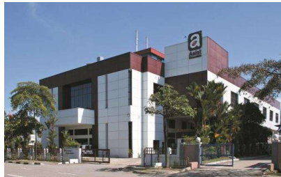
26 Tuas Avenue 7, Singapore
