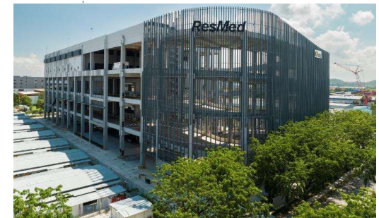
3 Tuas Avenue 2, Singapore
