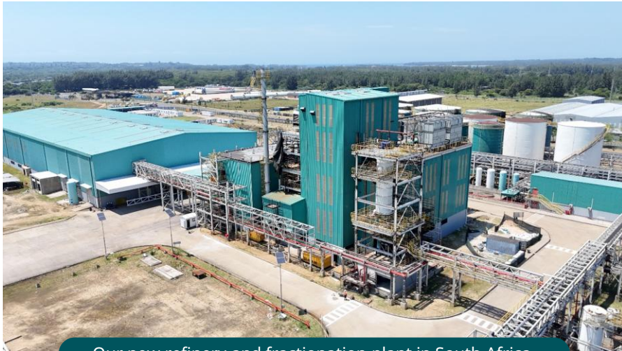
Our new refinery and fractionation plant in South Africa.
