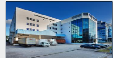
7 ALOG Changi DistriCentre 2 3 Changi South Street 3
