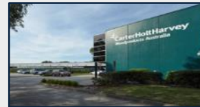
24 41 – 45 Hydrive Close, Dandenong South
