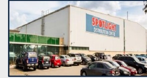
19 217 – 225 Boundary Road, Laverton North
