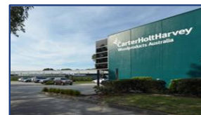
24 41 – 45 Hydrive Close, Dandenong South
