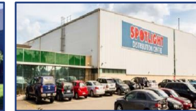
19 217 – 225 Boundary Road, Laverton North
