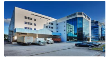
7 Cache Changi DistriCentre 2 3 Changi South Street 3
