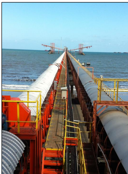
Figure 5:5 Barge loading conveyors at the BIB' Bunati Port
