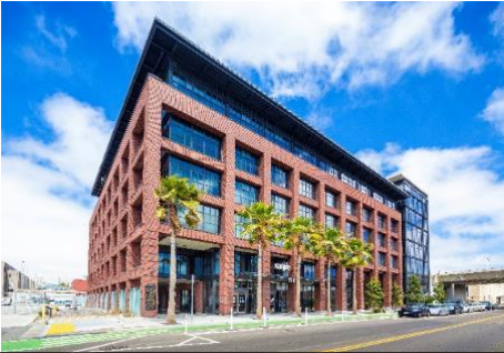
510 Townsend Street, San Francisco, US
