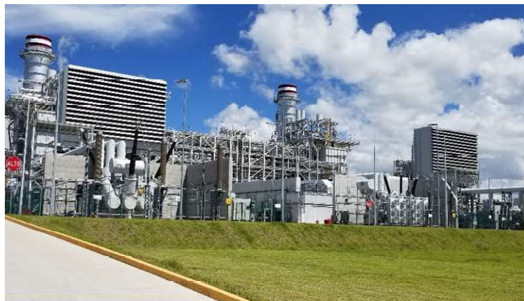
Figure 4-3: EVM II GSU and Air Inlets
