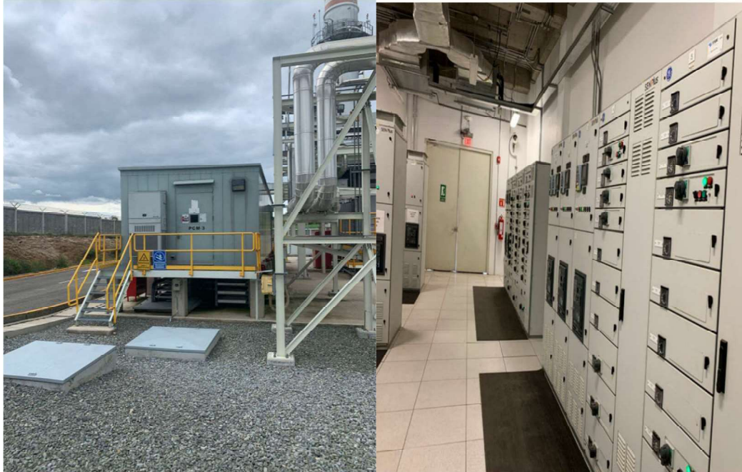
Figure 3-8 Power Control Modules
