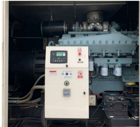
Figure 3-11 Emergency Diesel Generator
