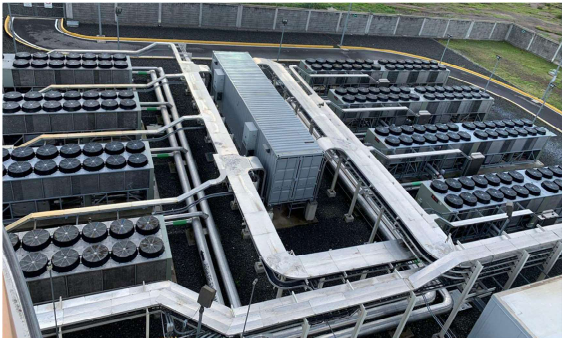
Figure 3-3 Chillers and Power Distribution Module
