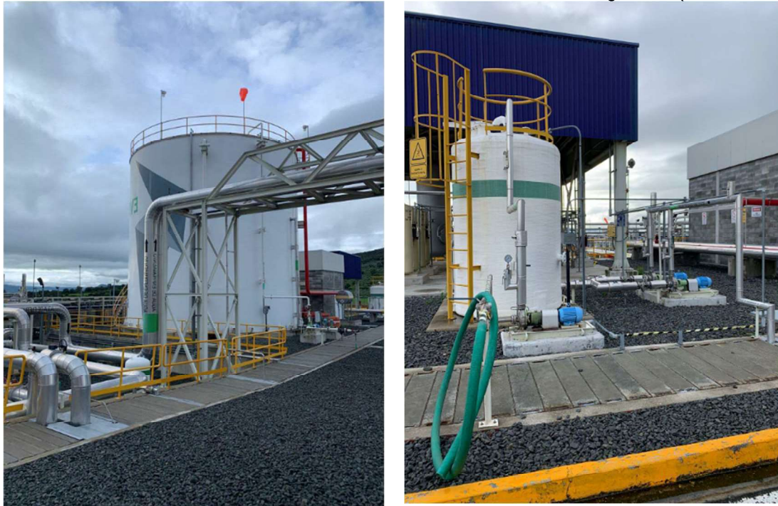
Figure 3-5: EVM I Demineralized Water Tank (right) and Service Water Tank (left)
