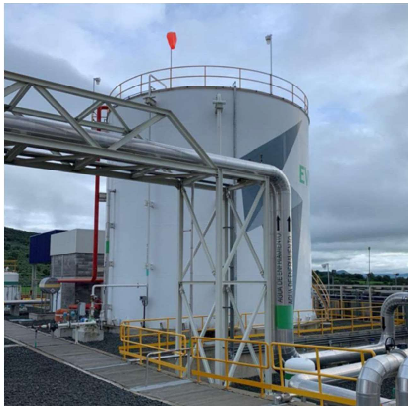
Figure 3-10: Service Water Tank
