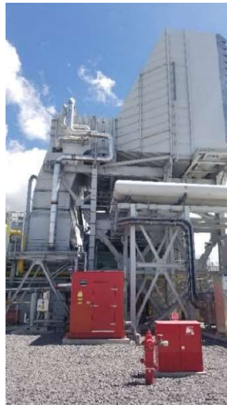
Figure 4-9: EVM II Gas Turbine Fire Protection
