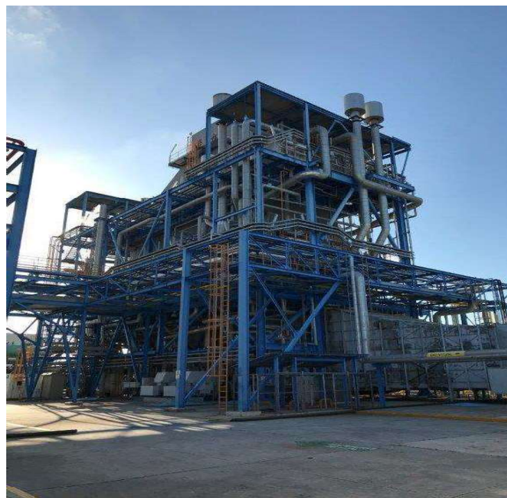
Figure 6-5: Heat Recovery Steam Generator at the Rio Bravo II Site
