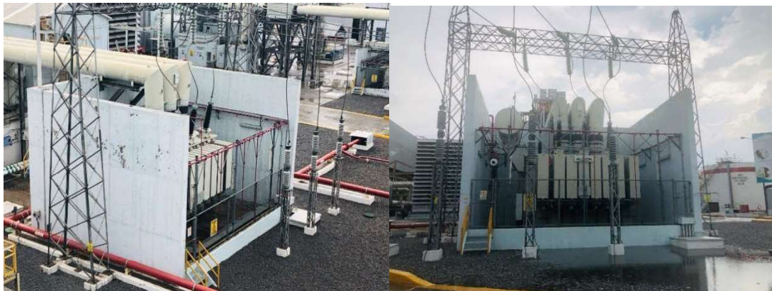
Figure 5-13: Steam Turbine GSU on Left and the Gas Turbine GSU on the Right
