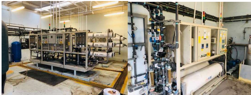
Figure 5-11: Water Treatment Plant Equipment
