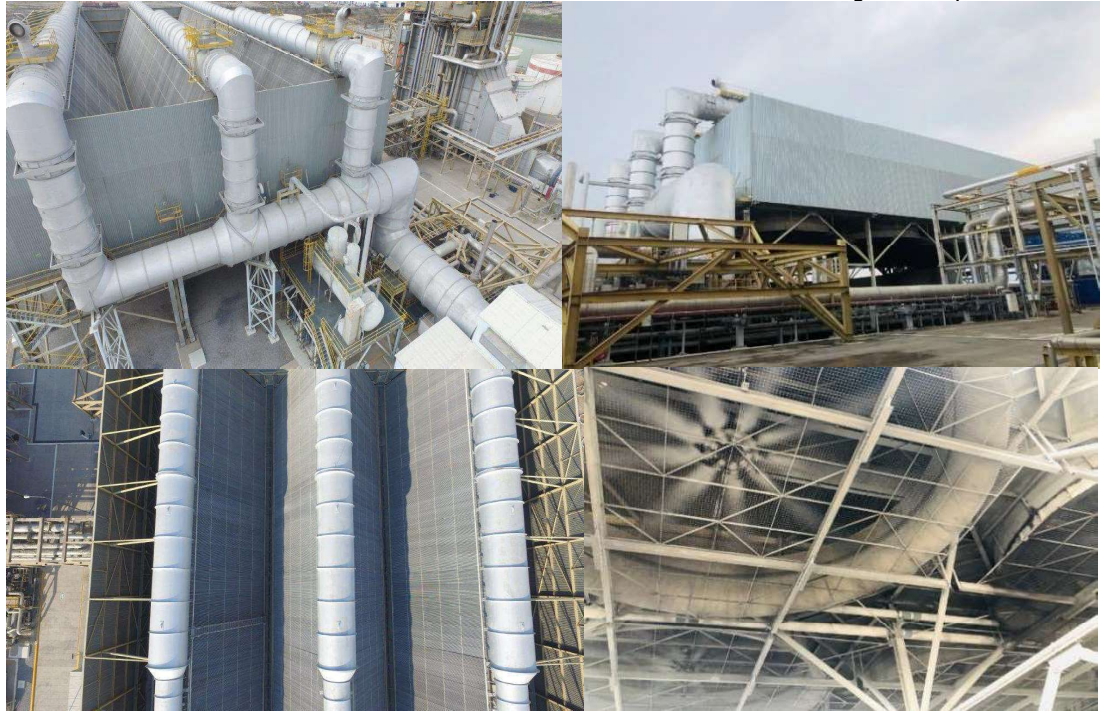
Figure 5-6: Air Cooled Condenser at Saltillo Site
