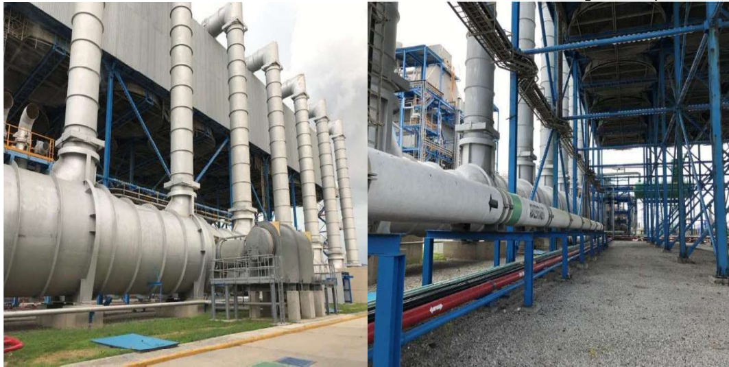
Figure 6-7: Air Cooled Condenser at Rio Bravo II
