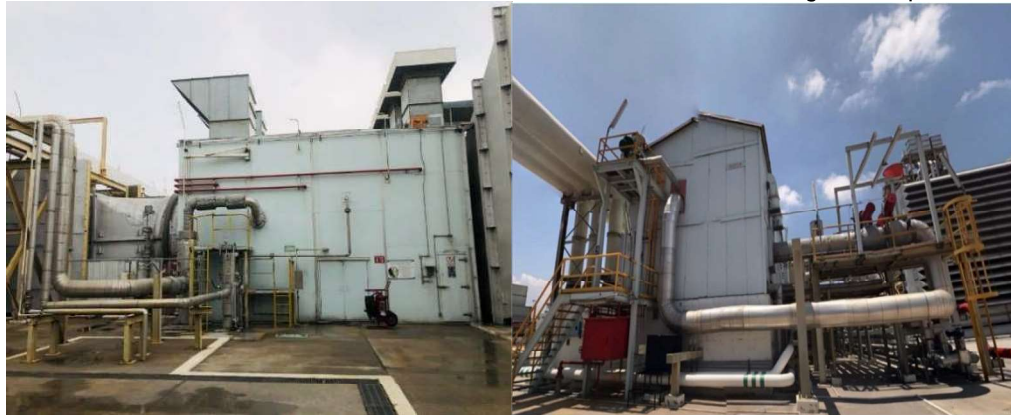
Figure 5-12: GT Generator Enclosure on Left and ST Generator Enclosure on Right
