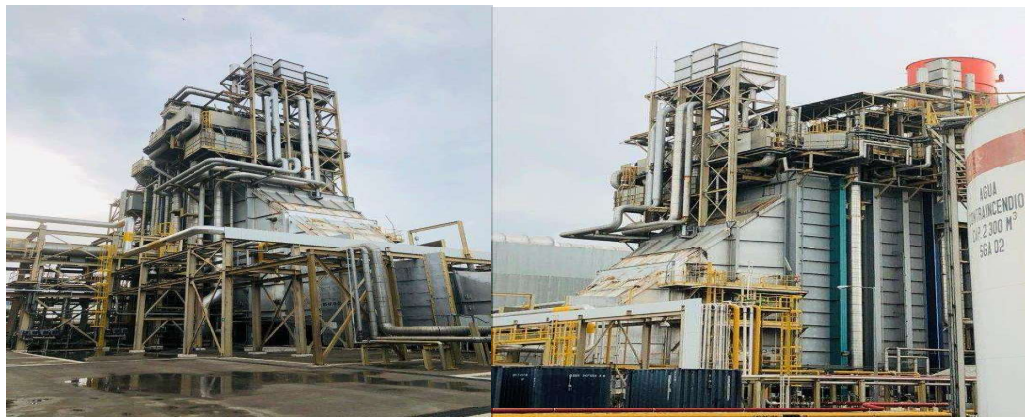
Figure 5-4: Heat Recovery Steam Generator at the Saltillo Site
