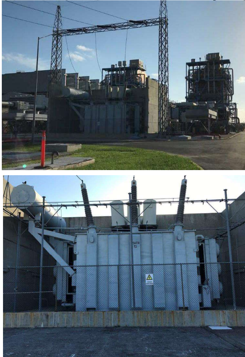
Figure 6-13: GSU Transformer at Rio Bravo II
