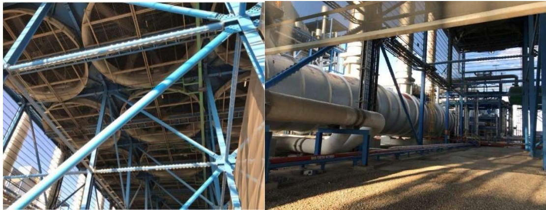
Figure 8-7: Rio Bravo IV Air Cooled Condenser
