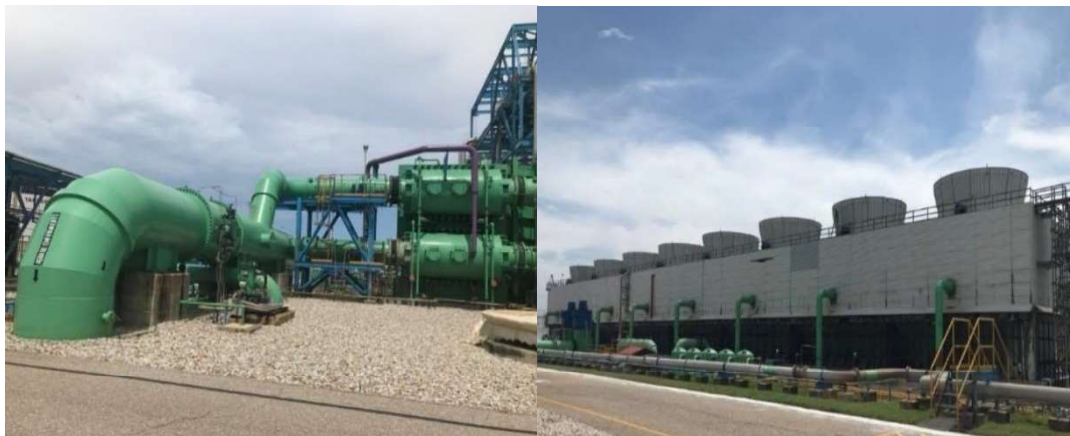
Figure 9-6: Condenser on Left and Cooling Tower on Right
