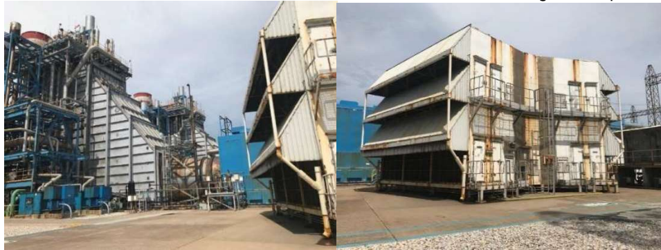
Figure 9-3: Altamira II Gas Turbine Exterior View with HRSG on Left and Air Intake on Right
