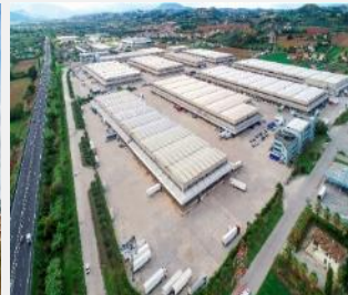
Centro Logistico Orlando Marconi Montepandone, Italy
