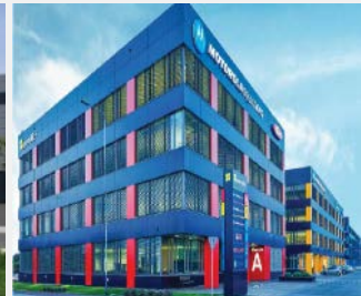
Green Office Kraków, Poland
