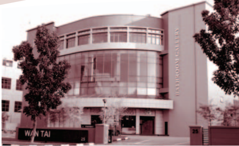
25 CHANGI SOUTH AVENUE 2
