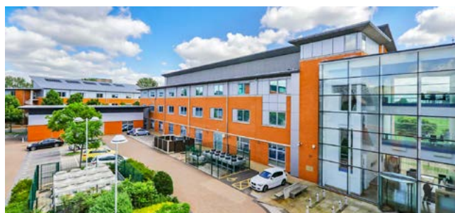
▲ Reynolds House (Data Centre)
