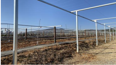
Scaffolding built with high standards
