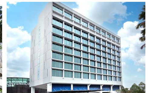
2 Changi Business Park Avenue 1 (Upcoming)
