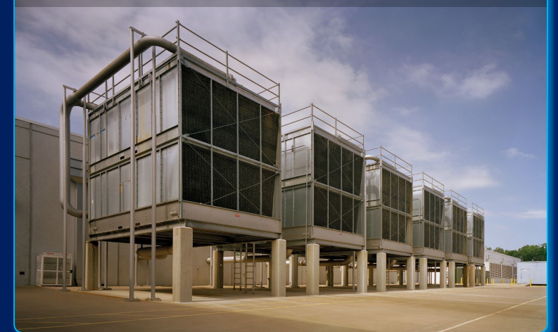
Concurrently Maintainable Chillers, Pumps and Cooling Towers
