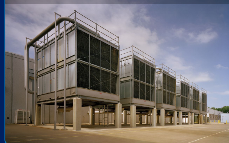
Concurrently Maintainable Chillers, Pumps and Cooling Towers
