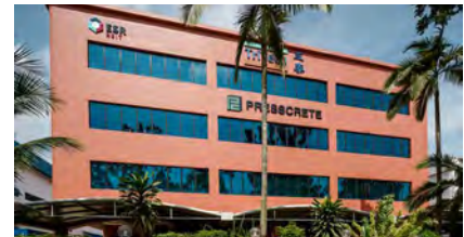
9 31 Changi South Avenue 2
