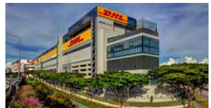
18 1 Greenwich Drive (DHL Supply Chain Advanced Regional Centre)
