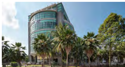
11 2 Tuas South Avenue 2
