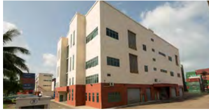
5 79 Tuas South Street 5
