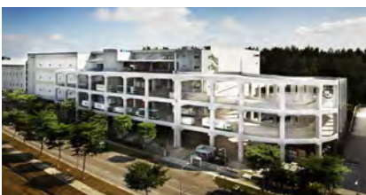
13 51 Alps Avenue (Schenker Megahub)
