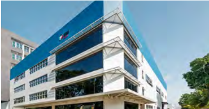
13 60 Tuas South Street 1
