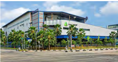
4 81 Tuas Bay Drive
