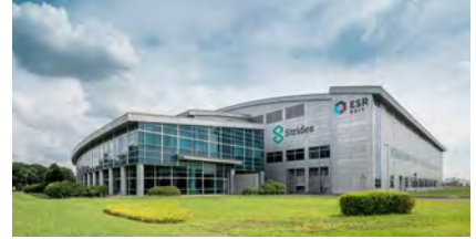
18 3 Tuas South Avenue 4
